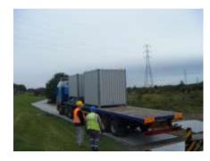
A series of track mats were used to provide a temporary access road to the concrete plinth, over the existing Type 1 track, to protect the site services beneath. These were removed after completion of the delivery lorry movements and crane activities.
