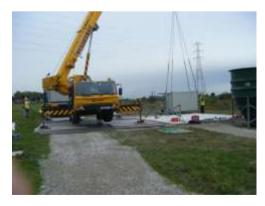
A 35te lorry mounted crane was used to off-load all the plant/equipment. The three parts of the Mobile HYRATE biofilter tower unit were assembled and positioned using the same crane.
