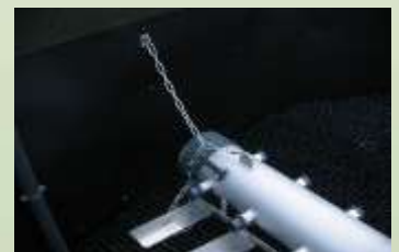
Distributor arms are fitted with Quick strip full flow washout end cup & stainless steel chain
