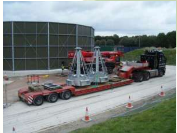
Delivery of HYCOVER Centre Columns.
