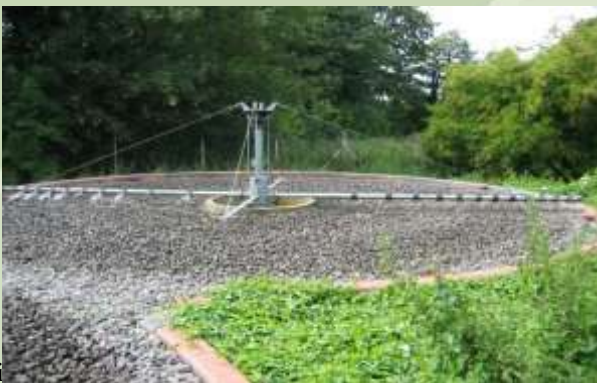
4 arm distributor in 12.0 mt dia HYRATE nitrifying filter.
