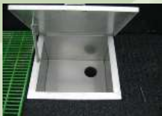
Stainless Steel washout box set into surface of media adjacent to access stairway
