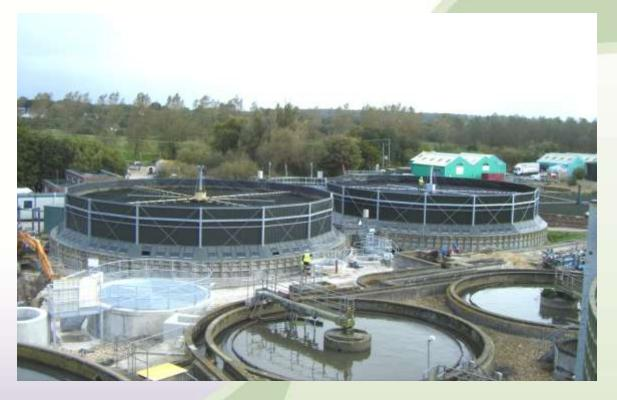
Space on site was at a premium on this sewage treatment works. So the twin 24.5 mt dia HYRATE Polytower biofilters, each packed with 1767 m3 modular plastic media, having a surface area of  $150 \text{ m}^2/\text{m}^3$ , and installed to a depth of 3.6 mts, were constructed inside existing stone trickling filter shells. This enabled accommodation of an increased hydraulic and boilogical load to the plant within the available space.
