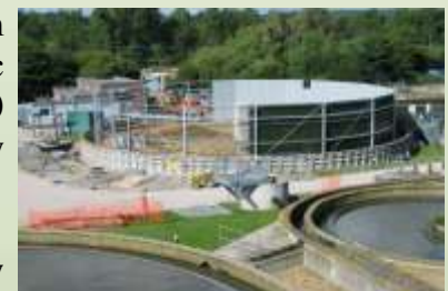
New 25 mt dia Polytower filter shell under construction using timber matrix as a working platform and for storage of materials.
