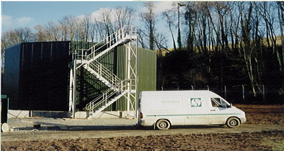
Sewaco design and build a wide range of HYRATE Polytower and Rectangular Biofilter shells suitable to contain plastic modular media with packed depths extending from 1.5 mts to 7.2 mts.
