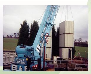
Typical installation of twin mobile HYRATE Biofilters providing temporary treatment of settled sewage effluent during refurbishment of existing stone trickling filters.
