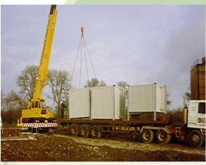
Modules are normally delivered to site on 40ft road transport, ready for immediate erection on flat concrete base slab.
